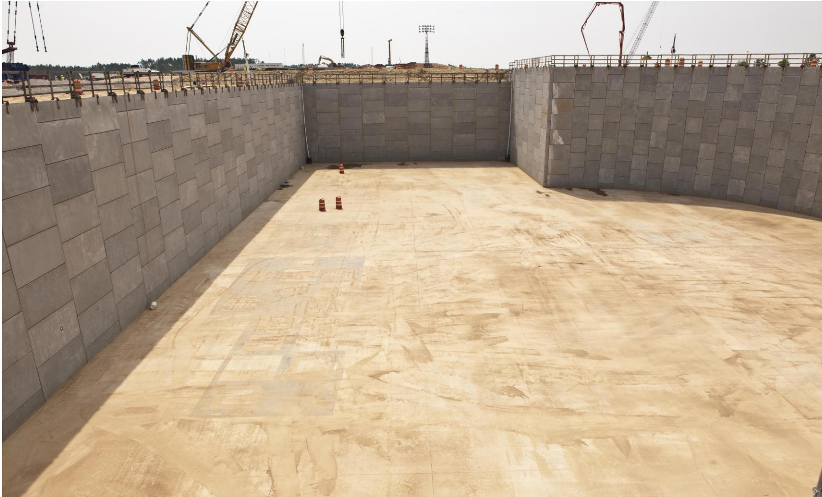
Vogtle Unit 4 nuclear island, prior to installation of basemat rebar
