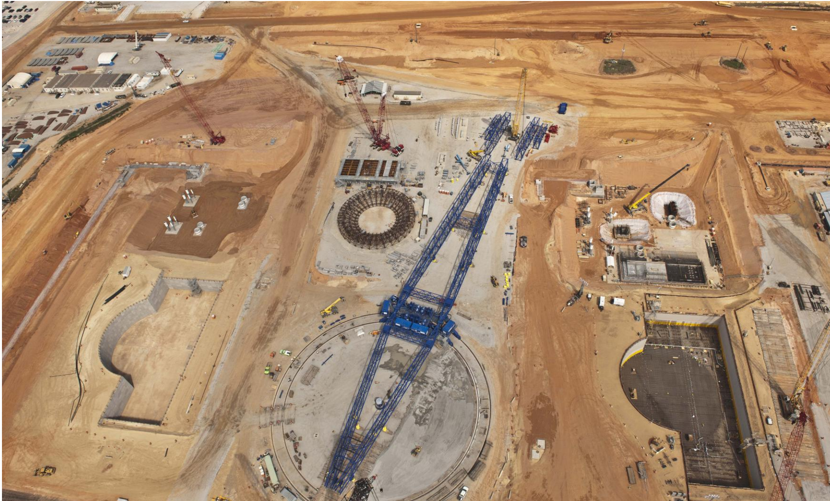
Assembly of large heavy lift derrick (blue) with Vogtle Unit 4 construction to the left and Unit 3 construction to the right.
