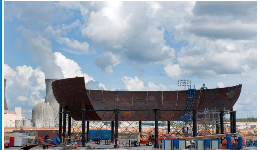
Vogtle Unit 3 containment vessel bottom head plates, after being fastened to assembly stand, are prepared for welding. September 21, 2011
